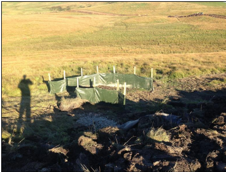
Plate 2: Typical silt traps
