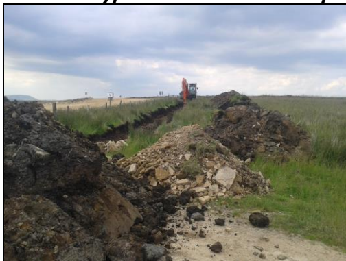
Plate 14: Typical overburden stockpile measures
