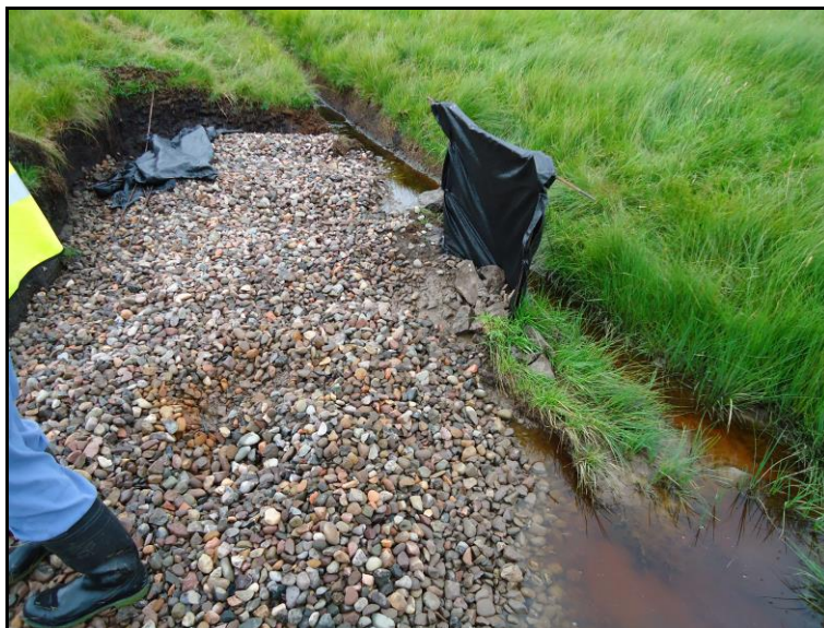
Plate 2: Typical silt traps
