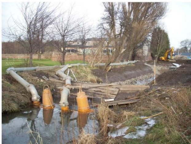
Plate 8: Full isolation – over pumping/siphon
