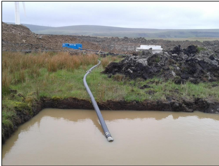
Plate 6: Typical 'Siltbuster' and settlement lagoon
