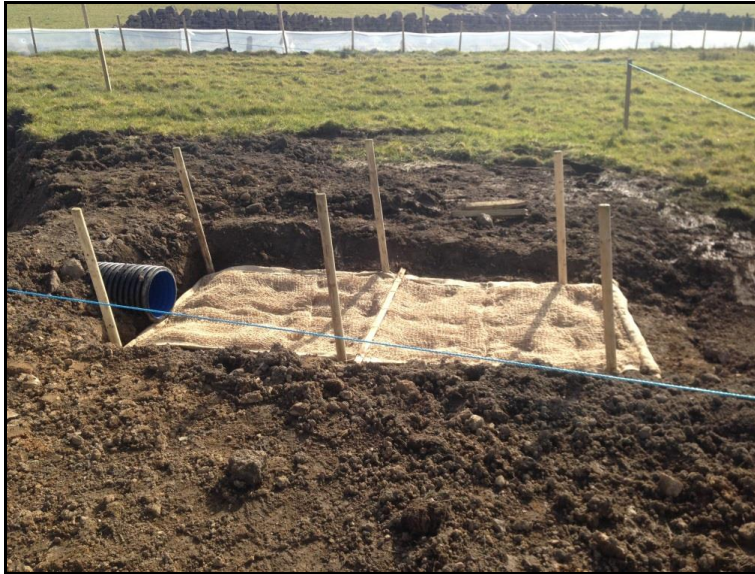
Plate 3: Typical silt mat to be placed at lagoon outfalls
