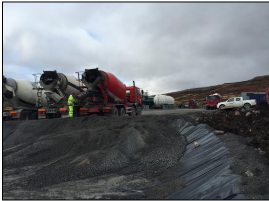
Plate 10: Typical concrete wash-out facility
