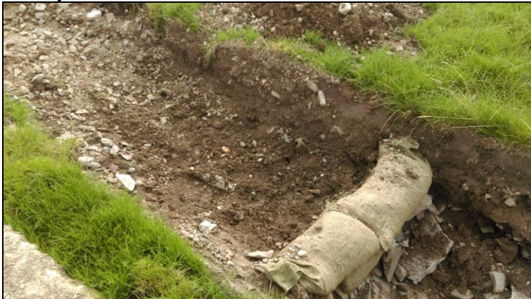
Plate 4: Typical check dams - to be installed in drainage ditches adjacent to the new spine road
